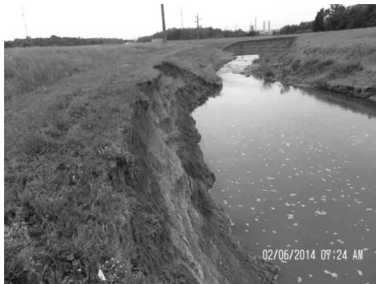
Figure 15. The view after dropping of riverbed after the flood;
